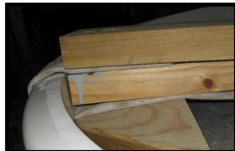
**STEP 5.** Use the predrilled holes in the lumber as a guide and drill through the top piece of fire hose in the correct location for the bolt. Use lumber to sandwich fire hose and hold it in place. Use caution. Threads from canvas fire hose can become caught in the drill making the drill and materials difficult to control. After drilling, enlarge the drilled holes in the fire hose by hand, if needed.
